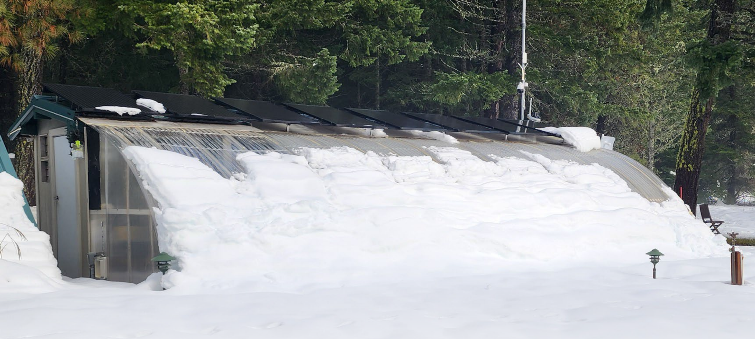
Solar-powered greenhouse with light snow load
